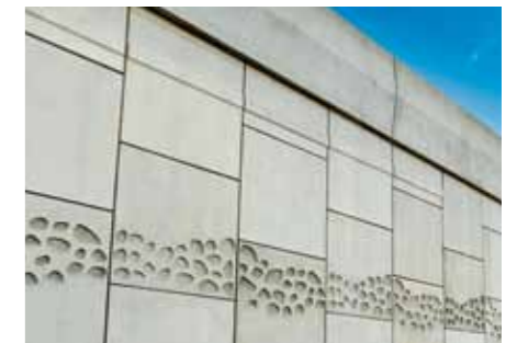
01-02-03 The architectural patterns applied to the 41 Reinforced Earth® walls supplied by RECo.
