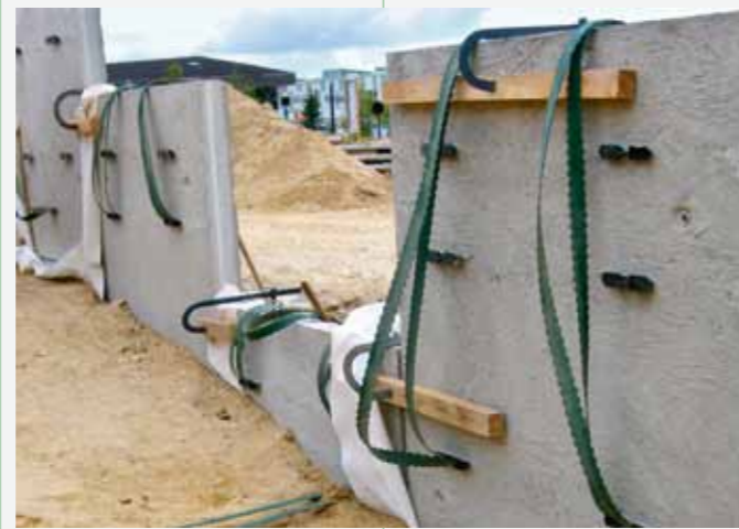
Facing panels equipped with GeoMega® connections and EcoStrap® reinforcements.
