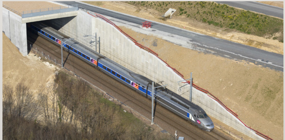
SEA high-speed rail project (France)
