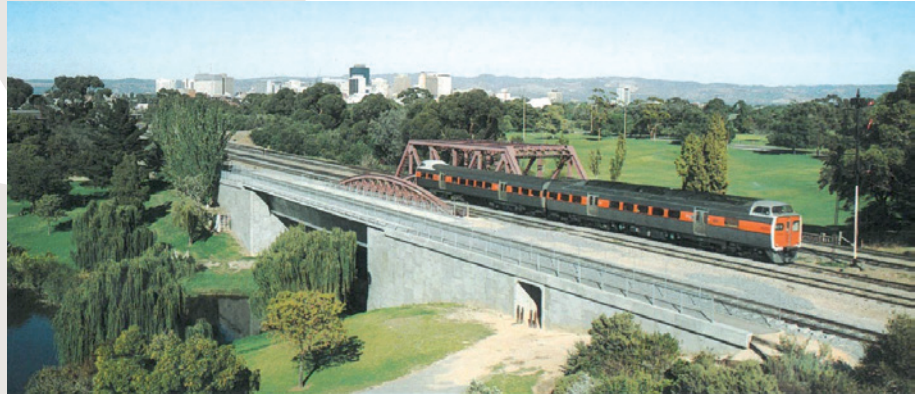
Torrens River bridge abutments - Australia (1982)
